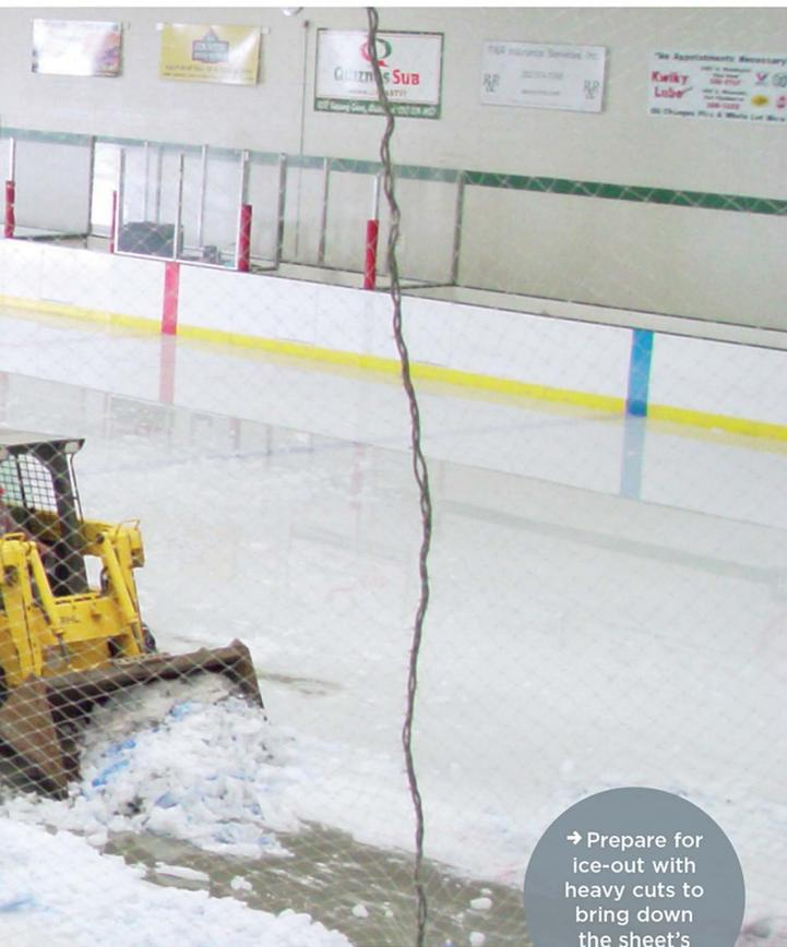
→ Prepare for ice-out with heavy cuts to bring down the sheet's thickness.
